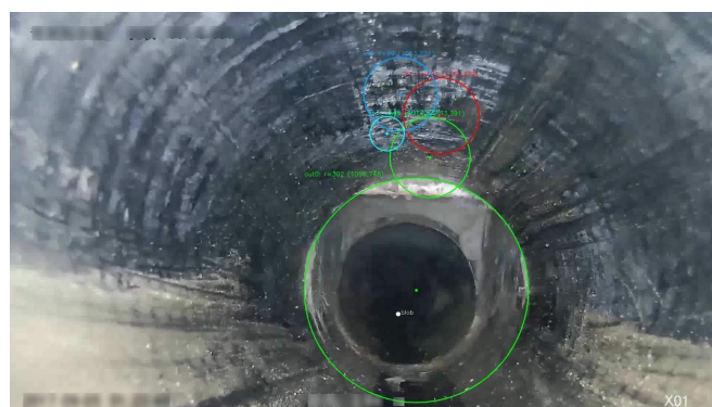
Figure. 1 Center detection on a QV-Pipe frame. The blue dot marks the detected pipe center; the green circle marks the estimated inner sampling radius r ; the red circle marks the estimated outer sampling radius R .
